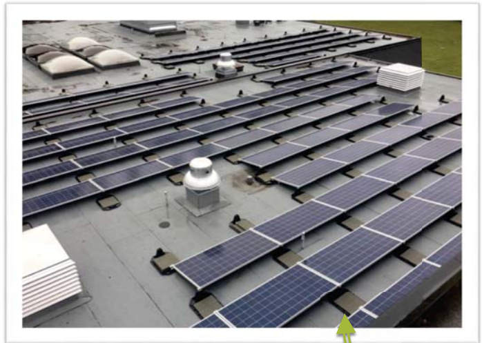
Solar at Pender Harbour Secondary
