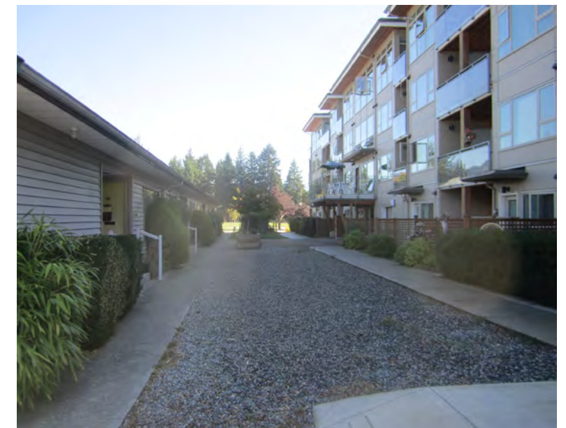
LANE BETWEEN BLOCK B & JACK NELSON BUILDING LOOKING EAST
