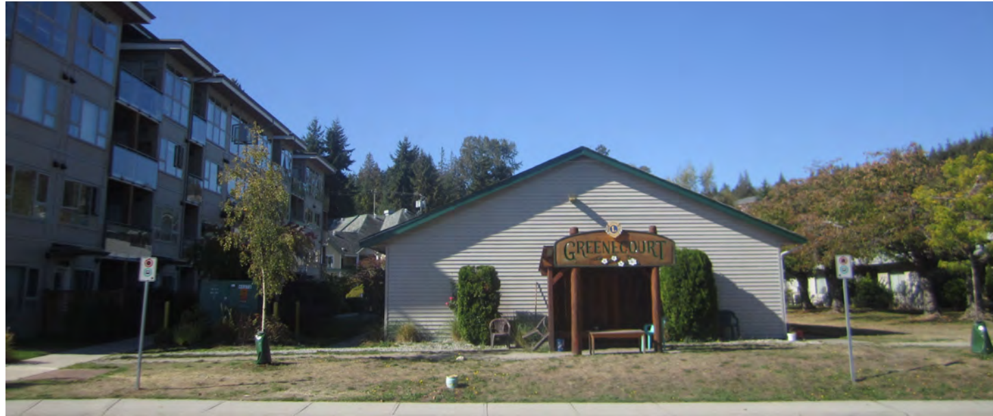
BLOCK B LOOKING WEST FROM OCEAN AVENUE
