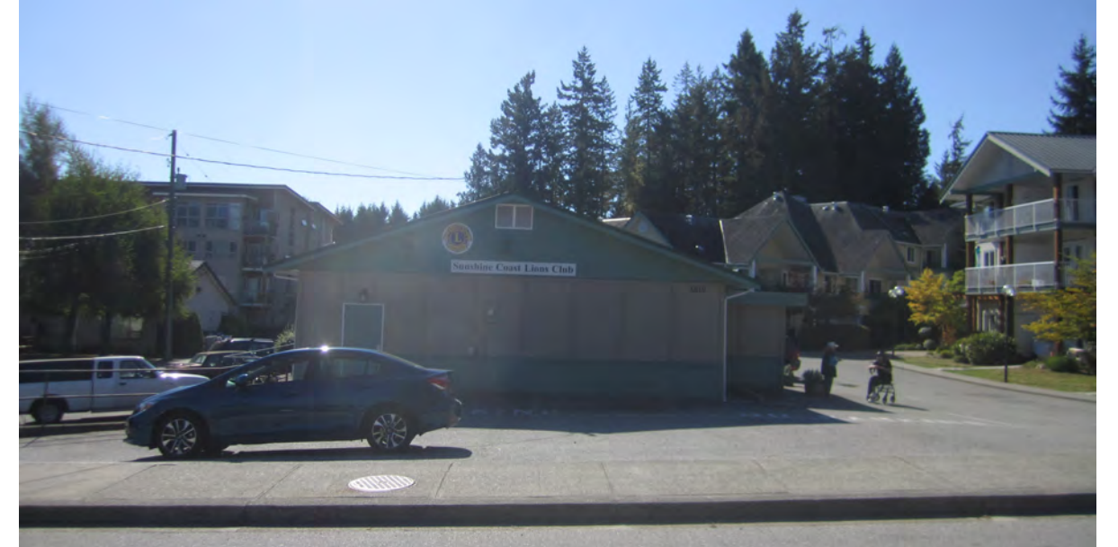
LIONS HALL, BLOCKS D & E LOOKING SOUTH FROM MEDUSA STREET
