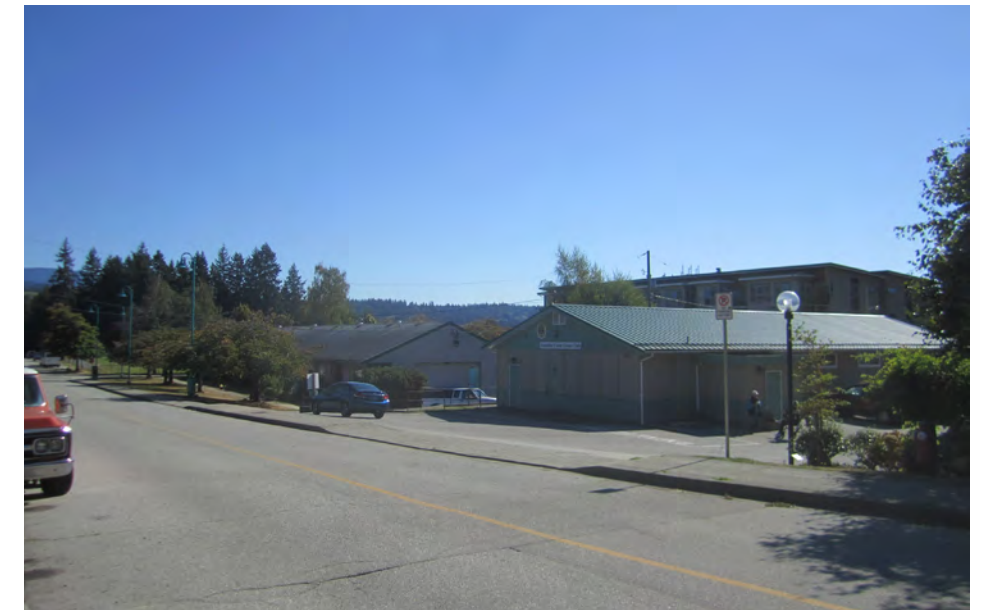
PROJECT SITE LOOKING SOUTHEAST FROM MEDUSA STREET
