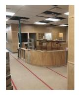
The upgrade for the StrongStart is near completion, with trim work and painting to be completed. Doorways and glazing have been reconfigured to ensure that the Tiny Town fits the new layout. A new fire alarm system, T-bar ceilings and emergency lighting will be completed soon and the expected completion date of this area is April 1. 2021.
