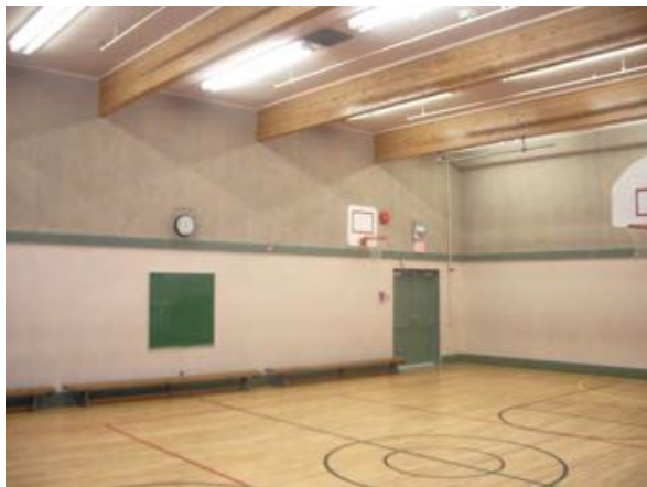
No. 3 –Gymnasium, which has no supply air ventilation
