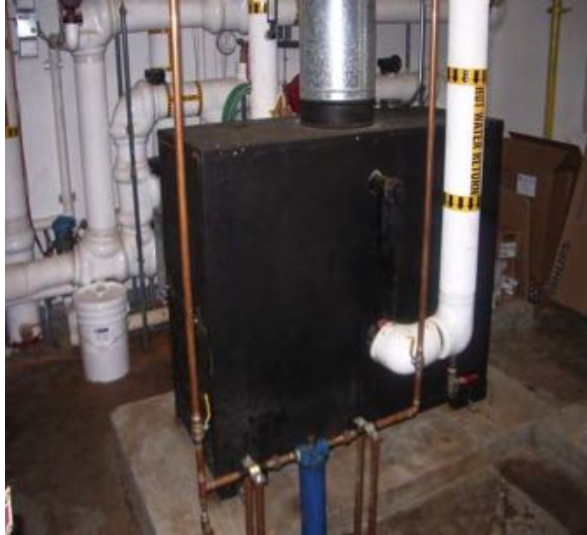
No. 1 – Parker propane fired boiler, which a standalone appliance providing heat to the school
