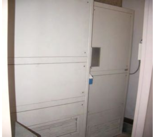
No. 2 – Temspec unit ventilators, installed in service closets with two units each, serving the Classroom and Library
